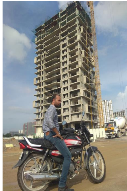
Safety Officer Mahammad Faruq stands in front of Myscapes building, Hyderabad
